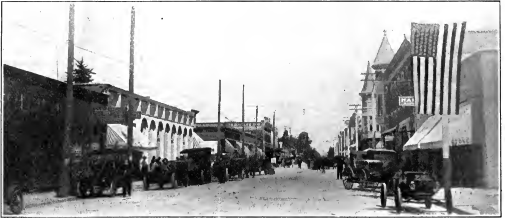
Looking North on Los Angeles Street, Anaheim.
